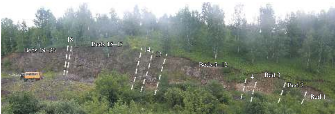
Fig. 6. Panoramic photo of section BS-091 in the roadside excavation along the left bank of an unnamed creek—a left tributary of Egos Creek, environs of the town of Prokopyevsk.
